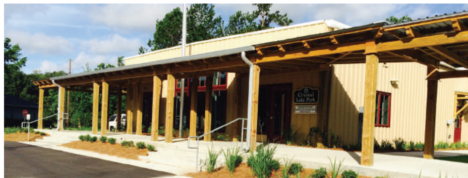
Moving to the new office located at 124 Lady's Island Drive on June 12, 2017.
